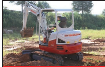
All Steel Construction
